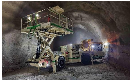
LIFTING AND INSTALLATIONS
